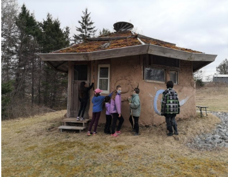
Exploring a cob structure at the Deanery
